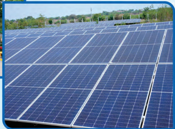
Installation of 1 MW solar power unit
